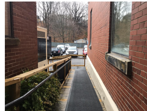
Back Entrance Ramp, Kentville Town Hall
