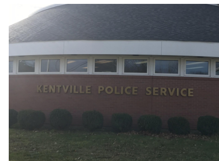
Police Station, Signage
