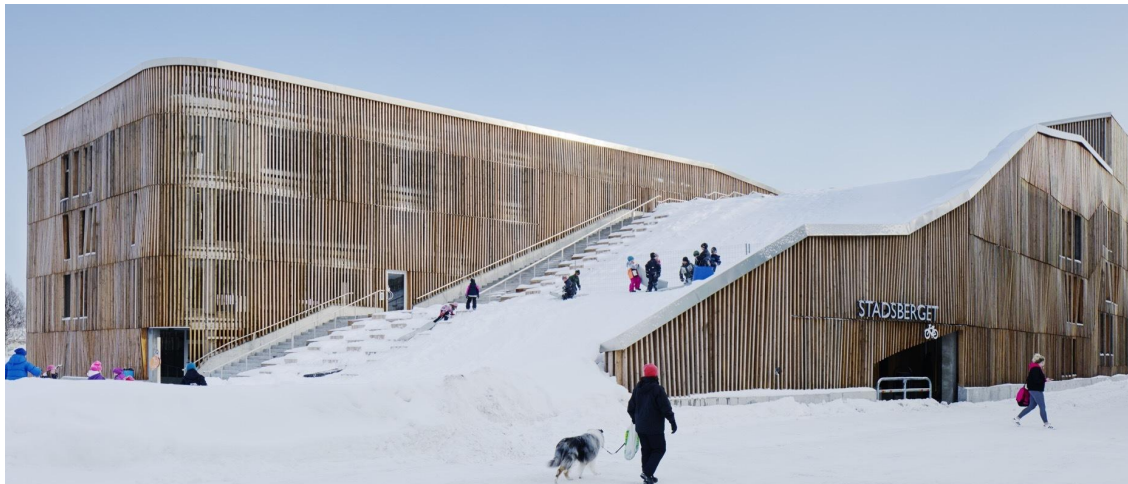
Parking Garage with Sled Slope, White Arkitekter + Henning Larsen Architects
