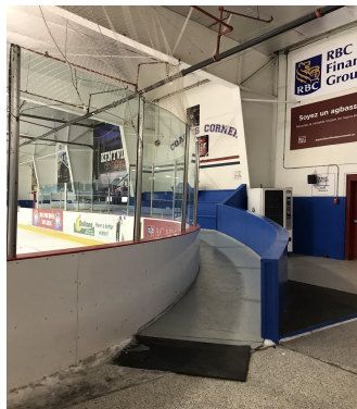
Centennial Arena, Ramp to Separated Accessible Seating
