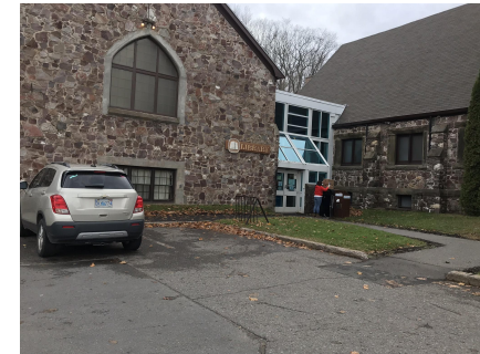
Kentville Library, Accessible Parking not near entrance
