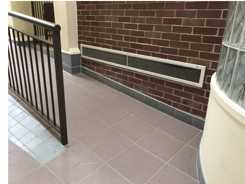
Interior Ramp, Kentville Town Hall
