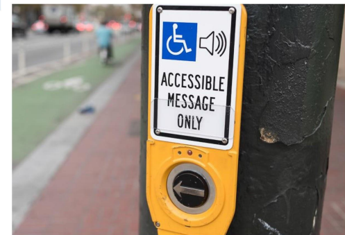
Top Detectable Warning Strip Bottom Audible Beaoning Accessible Pedestrian Signal
