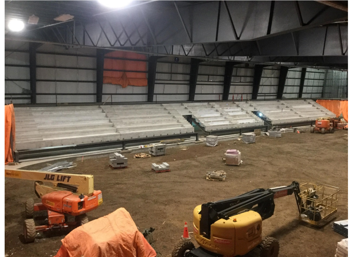
Mezzanine, Looking at rink stands
