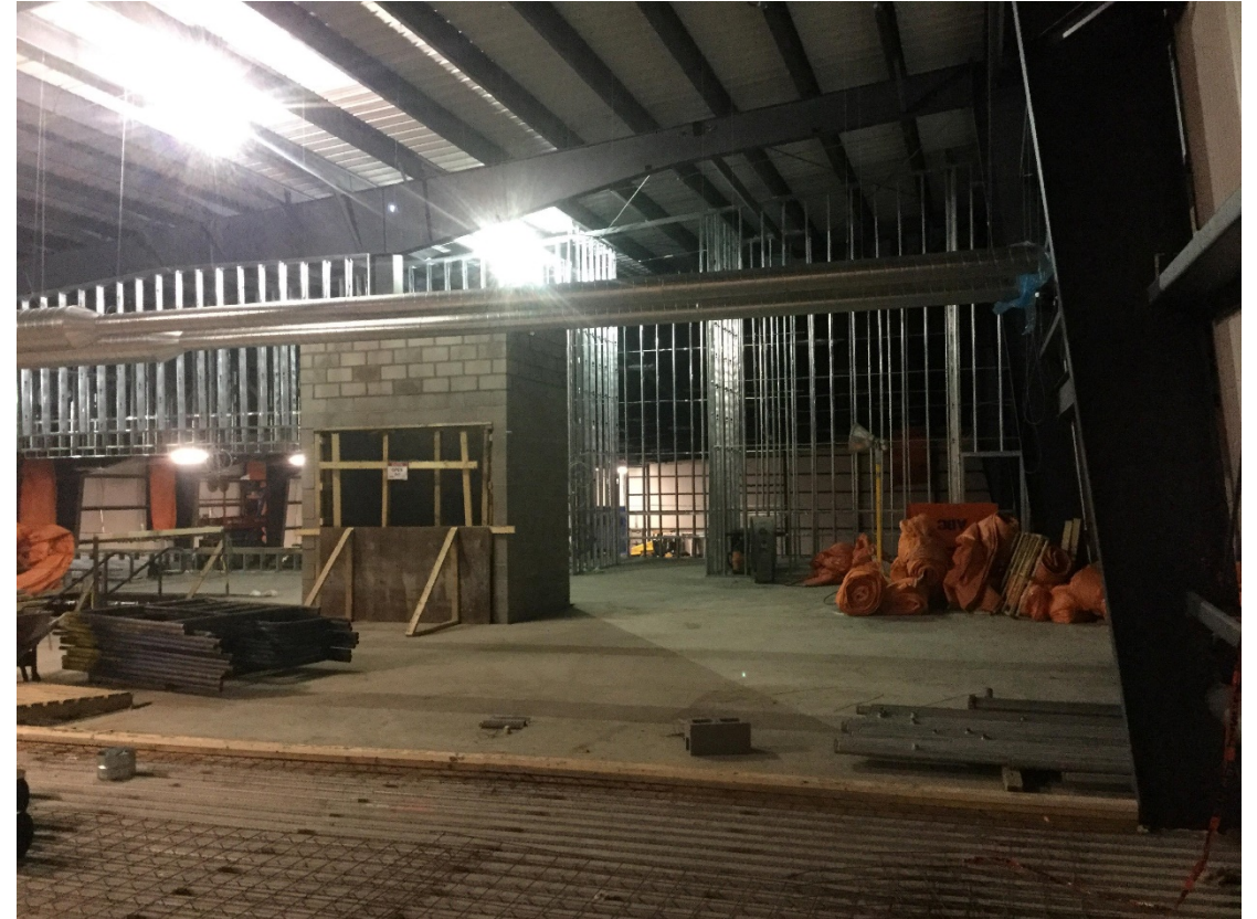
Mezzanine by rink stands, elevator and public washrooms behind it
