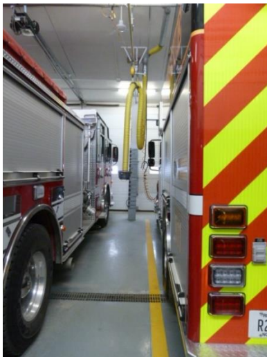
Doors are barely wider than trucks
