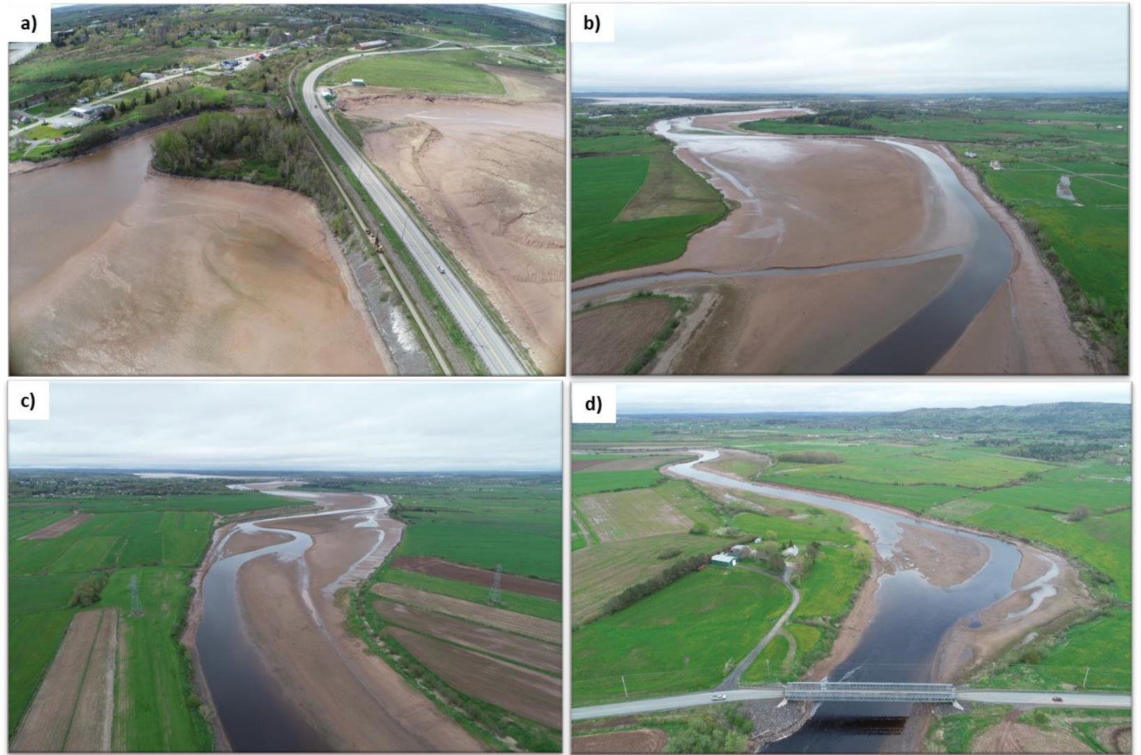
LOW ALTITUDE OBLIQUE AERIAL IMAGERY TAKEN ON MAY 23, 2019 BY GREG BAKER WITH DJI PHANTOM 4 RTK RPAS, A) CAUSEWAY AND TIDE GATE; B) LOOKING NORTH (DOWNSTREAM) FROM ALLEN BROOK; PHOTOS TAKEN MAY 27, 2019 AT C) LOOKING NORTH FROM HV TRANSMISSION LINES AND D) LOOKING NORTH (DOWNSTREAM FROM SANGSTER'S BRIDGE).
