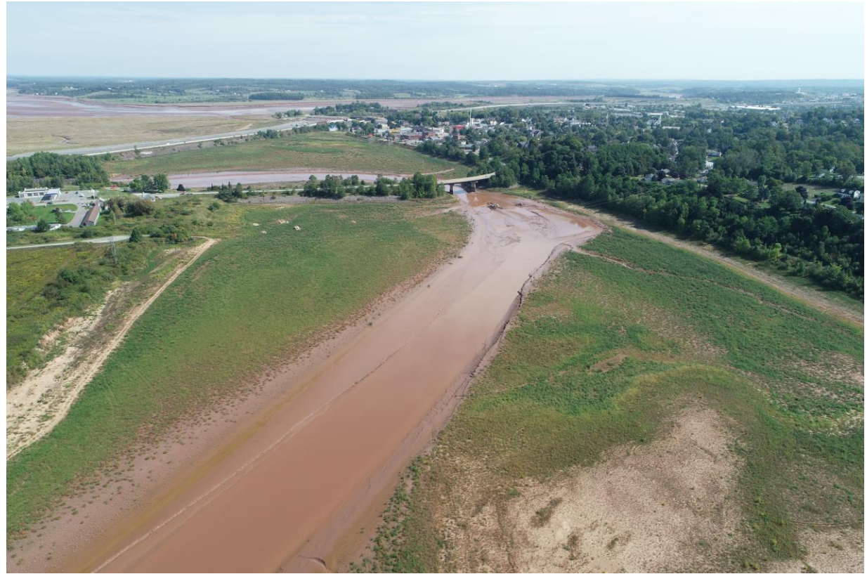
Upstream towards causeway Oblique aerial Sept. 12, 2022 – DJI Phantom 4 – CBWES Inc.
