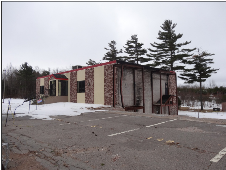
View facing Southwest from parking lot – former Legends Pub (part of Pine View Inn)
