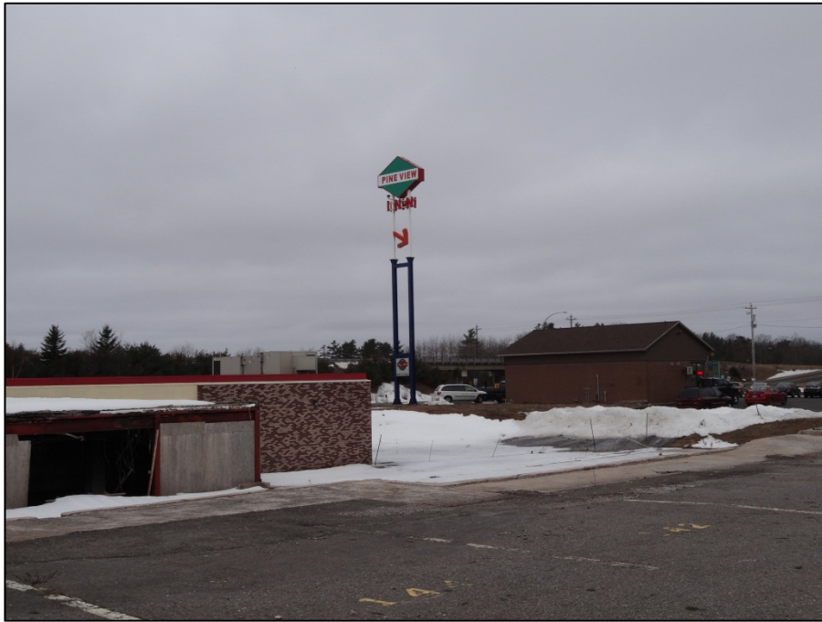
View facing Northwest from parking lot to Highway 101
