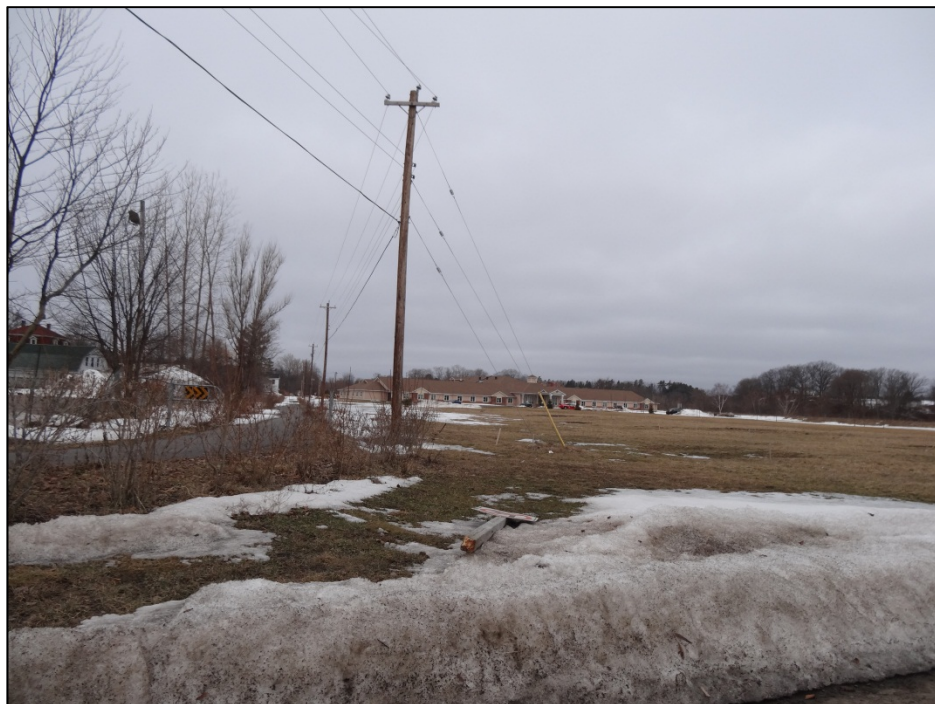
View facing Northwest at Webster St./River St. intersection
