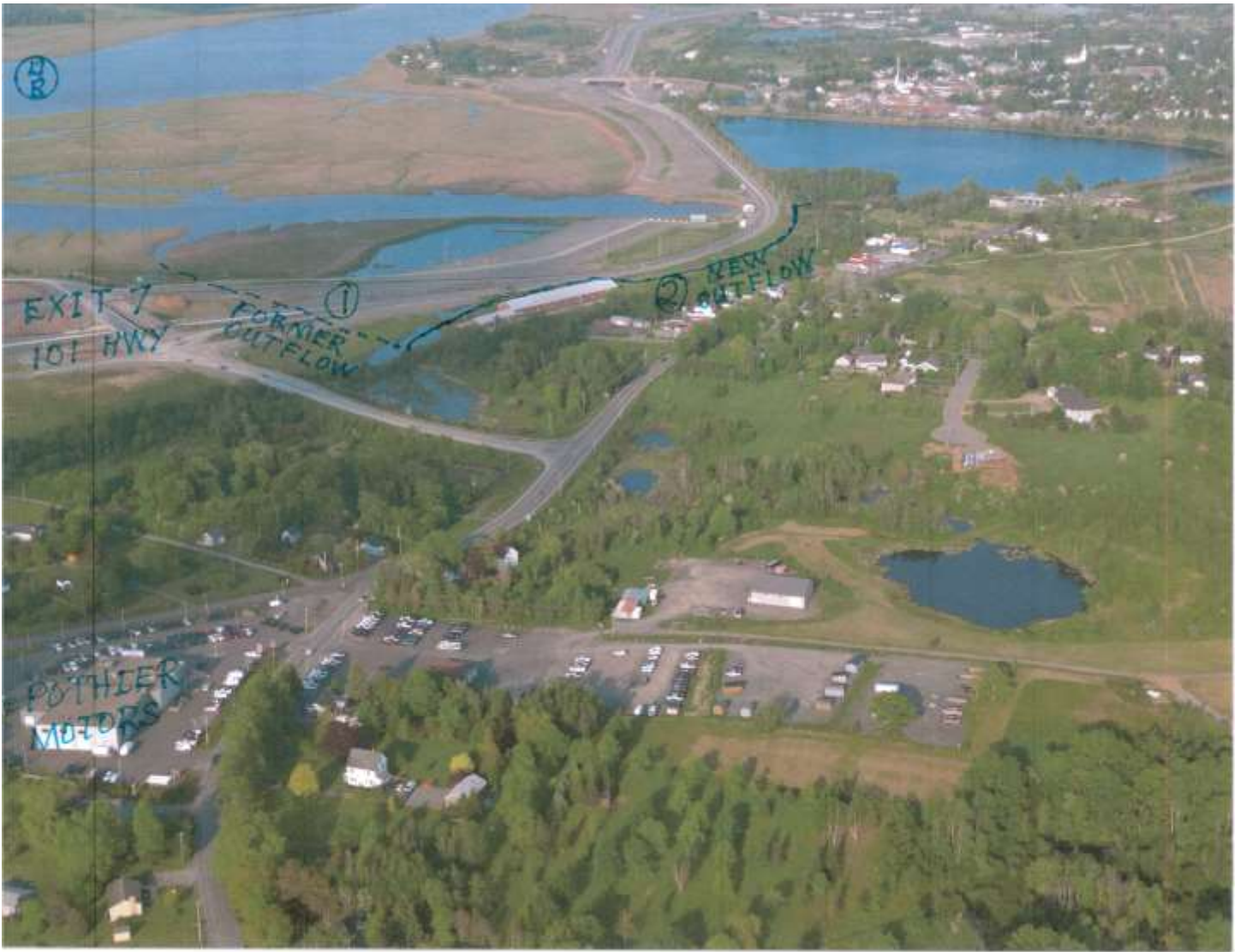
Picture #48 Former out-flow, #1 Present out-flow, #2
