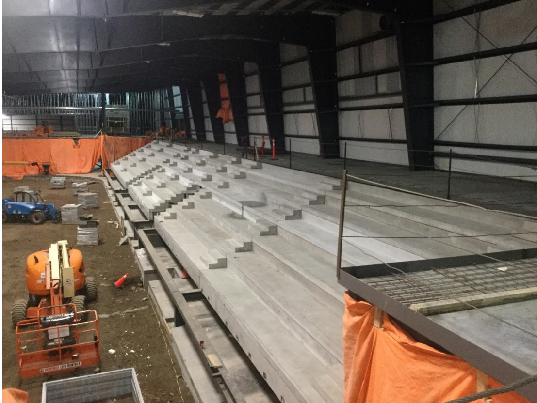
Mezzanine by mechanical room, looking at stands
