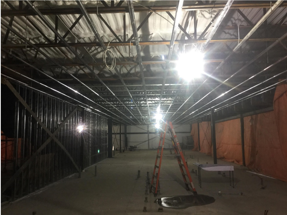
First floor center core, Fieldhouse dressing rooms
