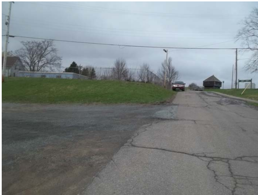
STREET VIEW LOOKING EAST ON FORT EDWARD STREET
