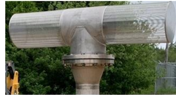
Figure 4.3: Pre Engineered Wedge Wire Intake screens. Tee style shown left image and S style shown in right image.
