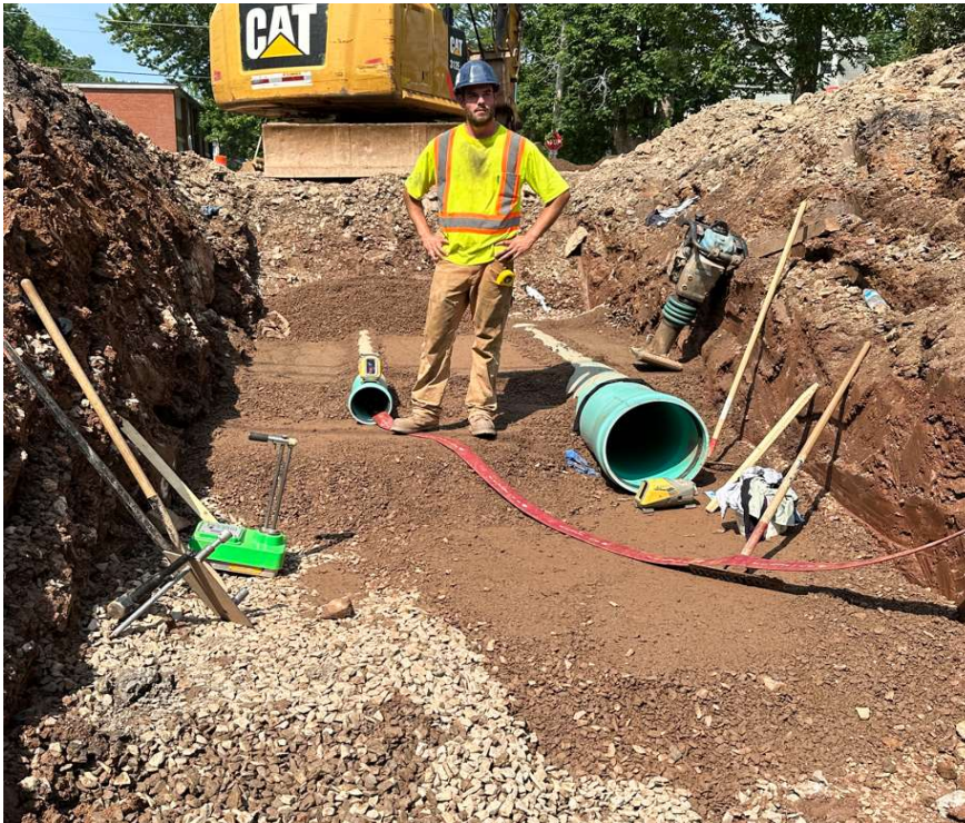
200mm sewer and 450mm storm installed with compacted type 1 gravel.
