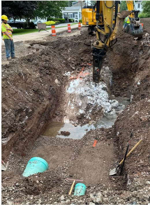
Rock breaking of gypsum ledge.
