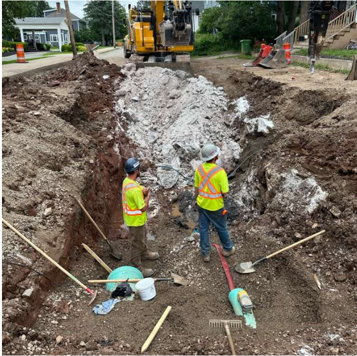
Rock breaking completed along the alignment.
