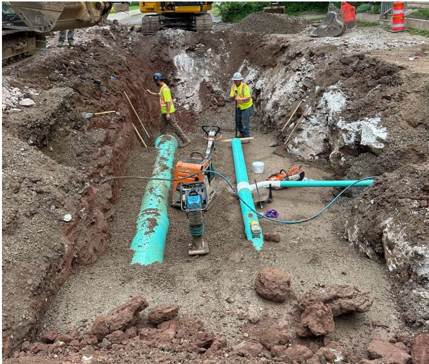
100mm sewer lateral installed to Civic # 420/422.
