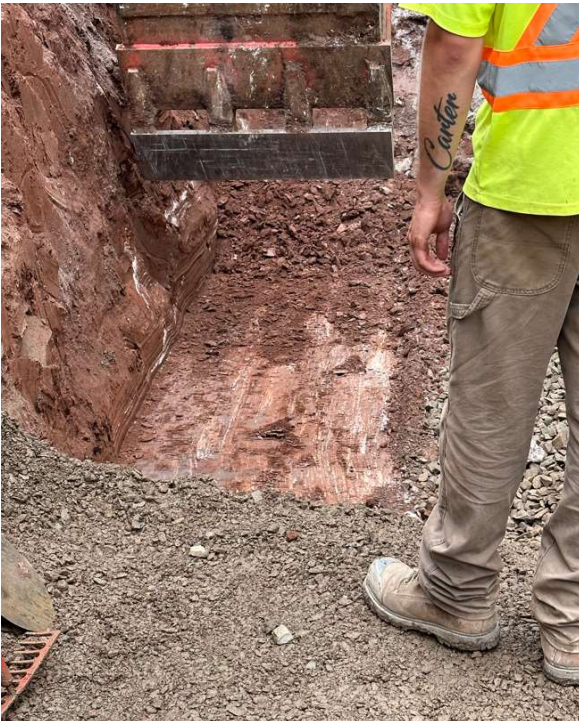
Undisturbed natural subgraded encountered at various along storm alignment.
