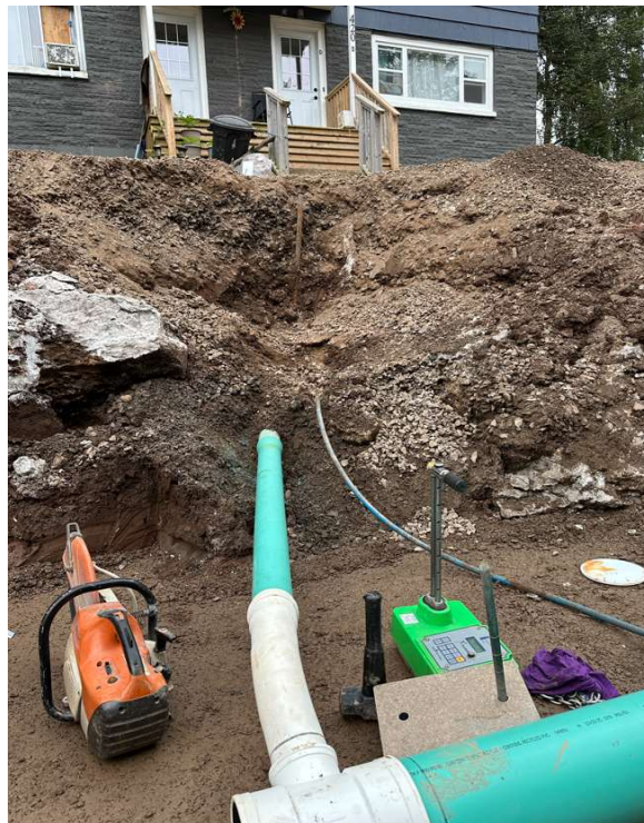
100mm sewer lateral installed to Civic # 420/422.
