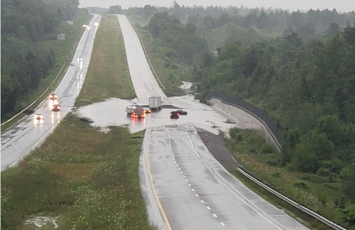
Hwy. 101 from Ellershous Overpass
