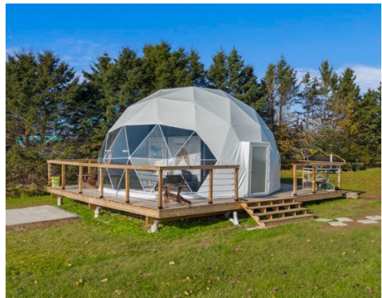
Photo 2: Proposed geodomes; photo taken from www.atlanticdome.com . Domes are to be placed on a wooden deck system as depicted with a sewer bed system for each dome.
