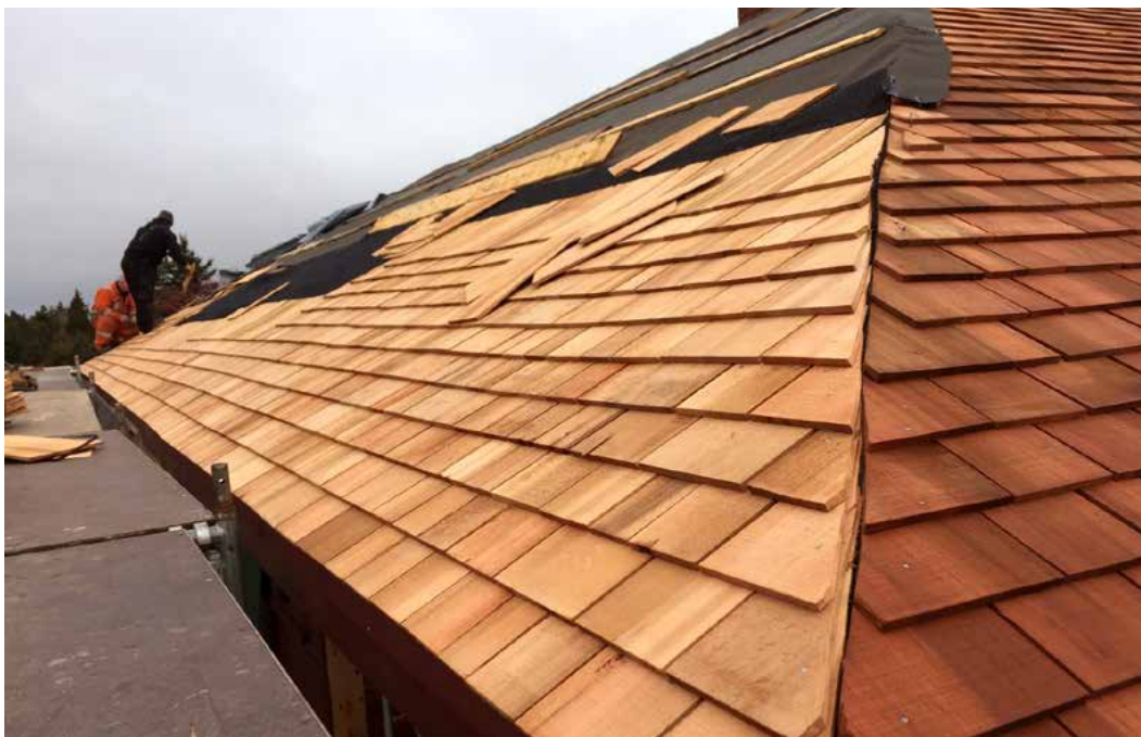
Restoration of Harbour Grace Railway Station Registered Heritage Structure, Harbour Grace, was completed in 2018 with support from Heritage NL. Perhaps the earliest purpose-built station in the province, the project saw the preservation of its original wood shiplap cladding and reinstatement of its historic wood roof.
