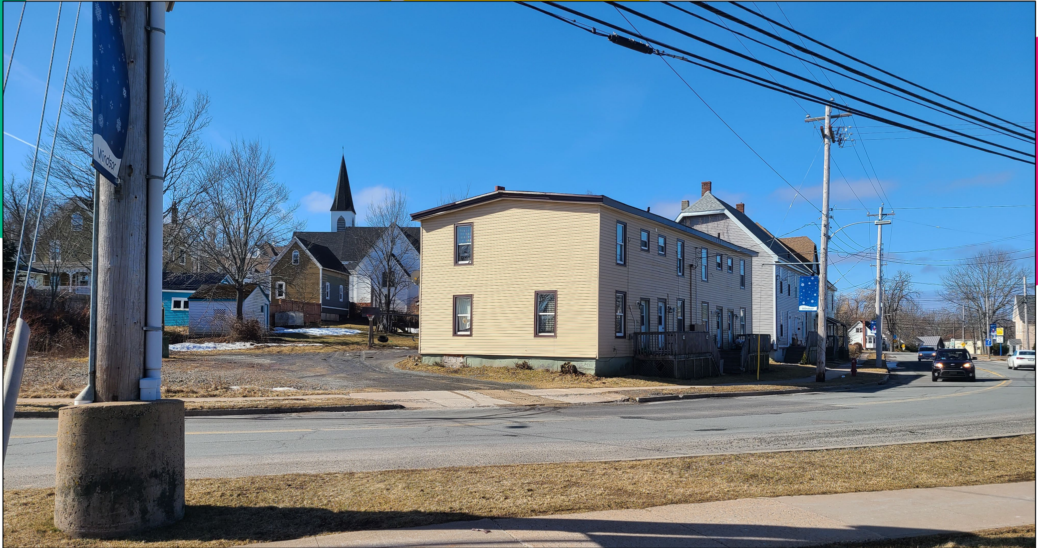
View of Subject Lot
