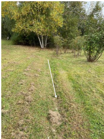
Shallow drainage ditch bordering right side of property; slope depicted by white arrow
