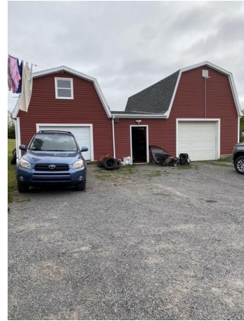
Close-up view of garage/motor vehicle shop
