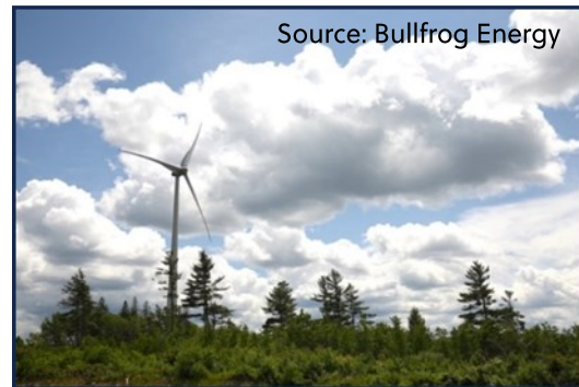
Figure 4: Ellershouse Wind Turbine
