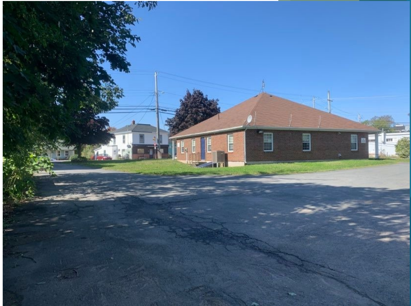
The rear of the building and the large parking area
