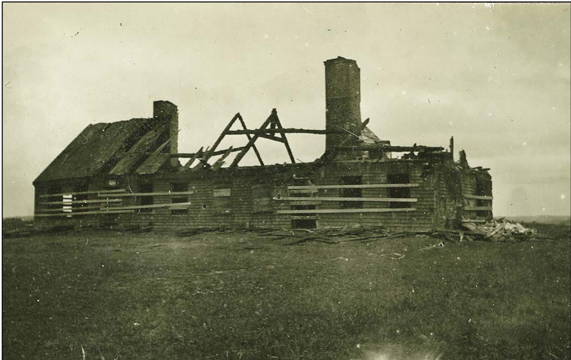
Figure 9: The burning of the 18 th century officers' quarters in progress (top); and the building in ruins (bottom) in 1923. SOURCE: NSA, Photographic Collection; NSA, Photographic Collection Acc. No. 7586.
