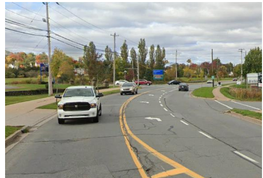
Figure 4 - Wentworth Road towards Payzant Drive
